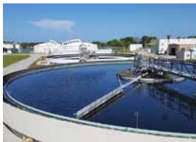
Station dessalement Safi
