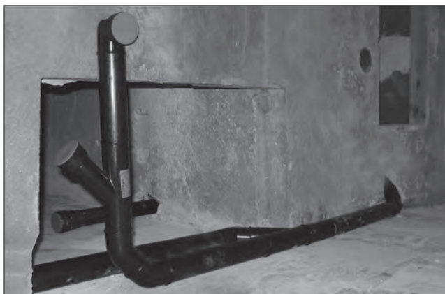
Illustration 9.2 Prefabricated pipe sections installed on site
